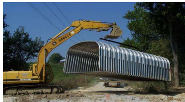
Lift and set in place
